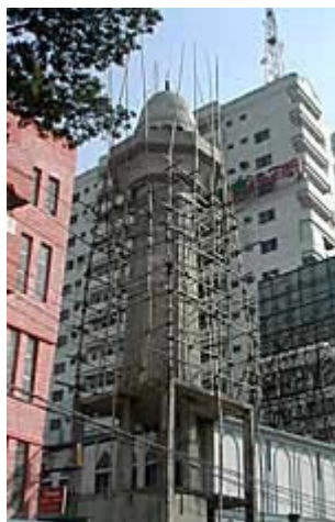
Project under construction
